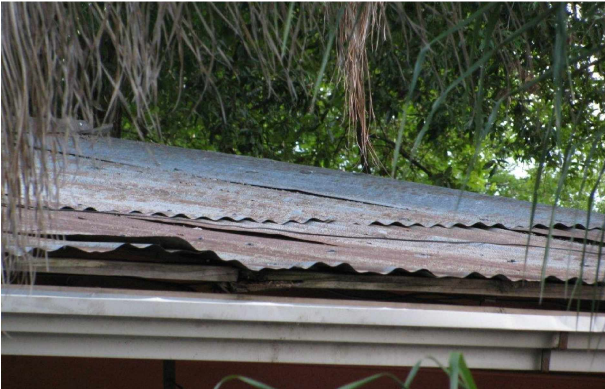
The Roof of the Dining Hall
